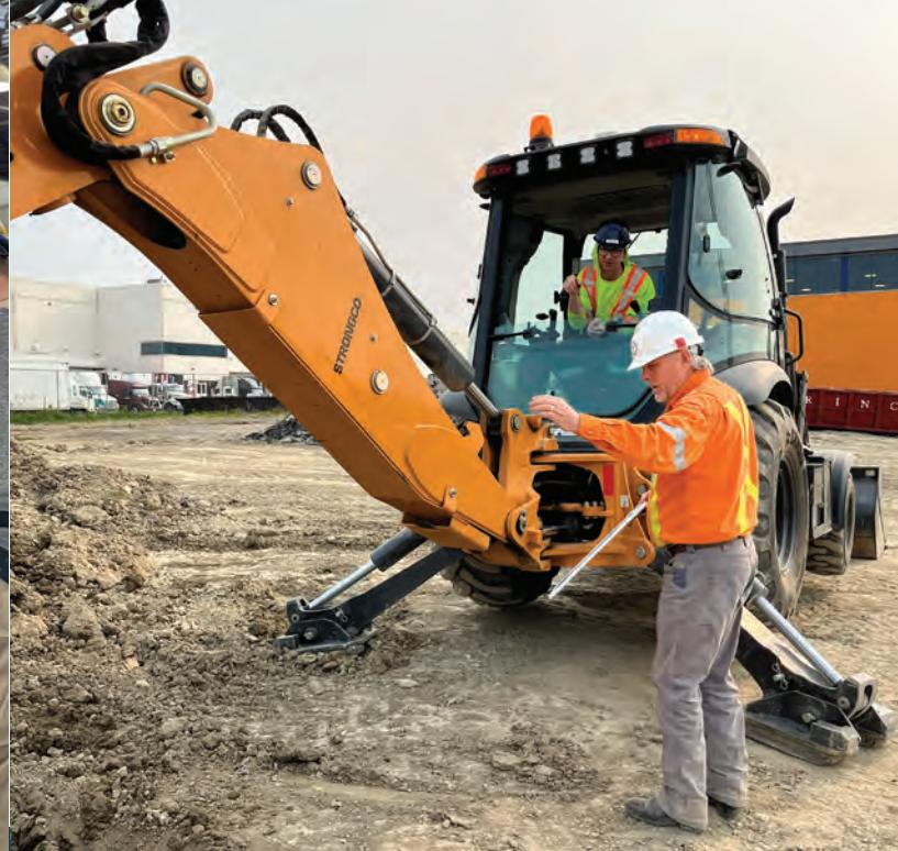
**A Tractor Loader Backhoe Operator inspects, maintains, transports, and operates full (standard) size equipment in the construction and industrial sectors. Some of the duties include performing a pre-operational inspection, transporting equipment, installing attachments, and loading and unloading equipment. In addition, operators will also work on excavating, trenching, grading, stockpiling and backfilling, among other duties.**
