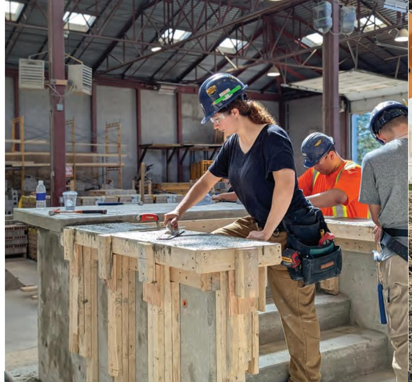
**Some of the tasks completed by a CCW trainee include constructing and dismantling concrete forms, scaffolding, ramps, catwalks, shoring, and barricades required at construction sites. In addition, they may mix, pour and spread materials such as concrete and asphalt. They may also assist with demolition, removal of rubble and other debris from a site and may operate various power tools, machines, and other equipment as directed.**
